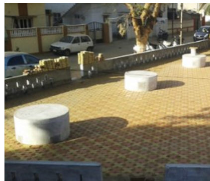
Flood control through GW recharge for housing colonies
